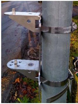
Figure 10: support & clamps, side view
