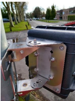
Figure 20: -45° orientation screw
