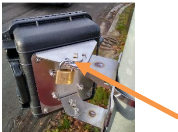
Figure 23: insertion space for anti-theft padlock
