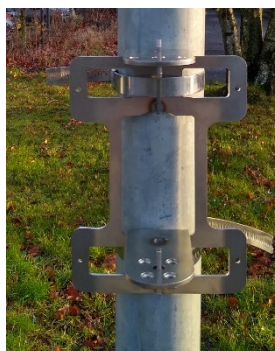
Figure 11: support & clamps, front view
