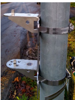
Figure 10: support & clamps, side view
