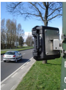
Figure 9: radar installed on the pole bracket
